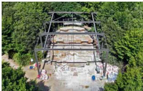
Setting up a bridge crane © Palace of Versailles, T. Garnier
