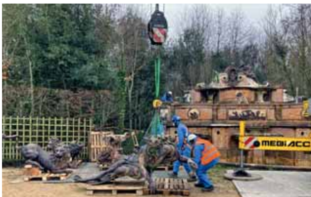
Removing the lead ornaments © Palace of Versailles, J. Camus
