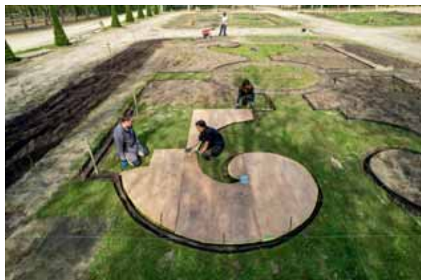
Working with jigs to replicate the parterre's scroll design ©Palace of Versailles, T. Garnier
