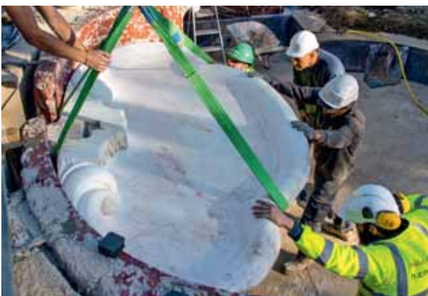
Refitting the central marble bowl © Palace of Versailles, D. Saulnier
