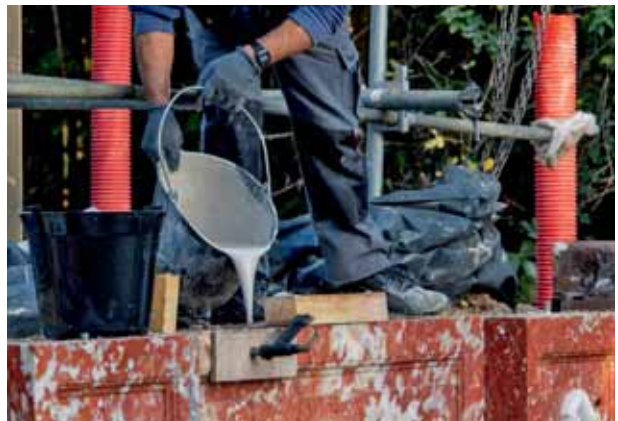
Limewash grouting between the stone and marble © Palace of Versailles, D. Saulnier
