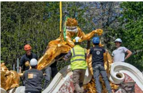
Refitting the restored lead ornaments © Palace of Versailles, D. Saulnier
