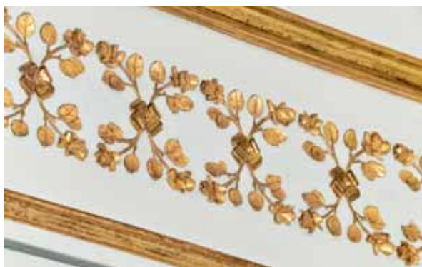
Detail of the cornice in the Méridienne Room © Palace of Versailles, T. Garnier
