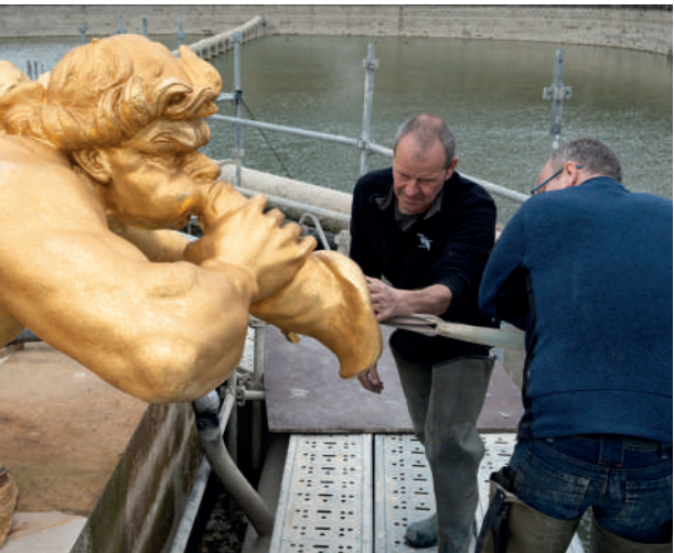
Installation of a new nozzle on a triton © Palace of Versailles, T. Garnier
