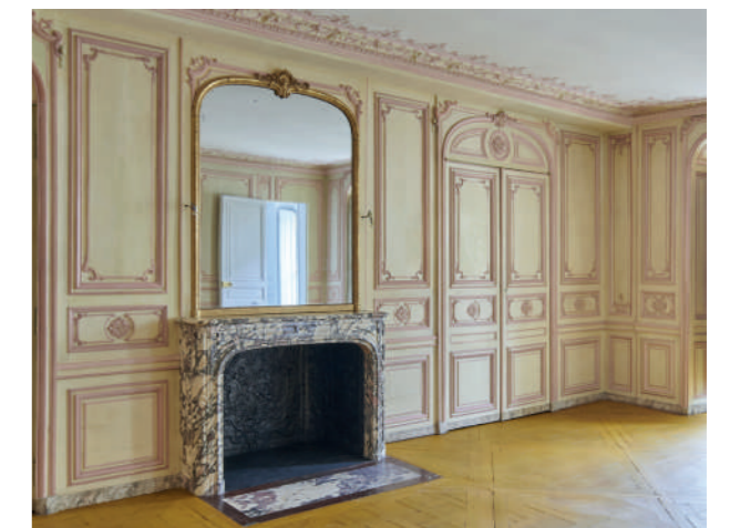
Buffet room after restoration © Palace of Versailles, C. Fouin
